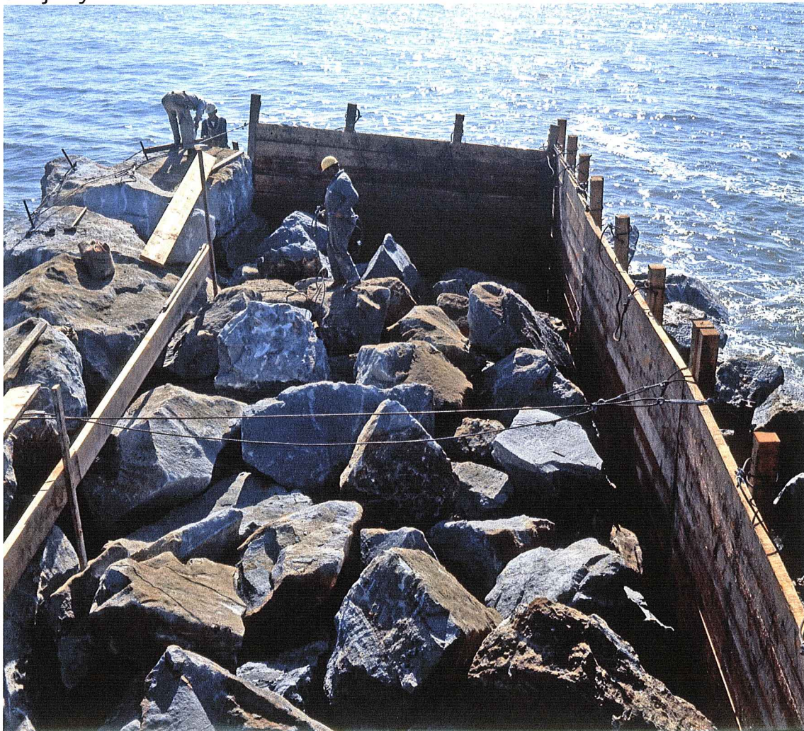
Figure 25. Beginning construction of the spine.
