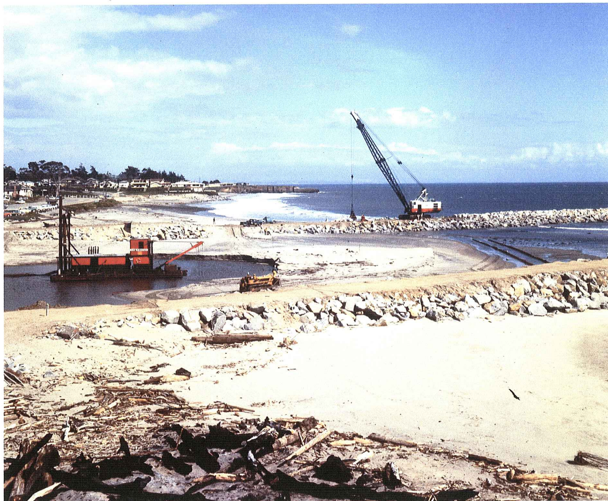
Fig. No. 8. Dredge digging out the beach to open the channel, the first time.
