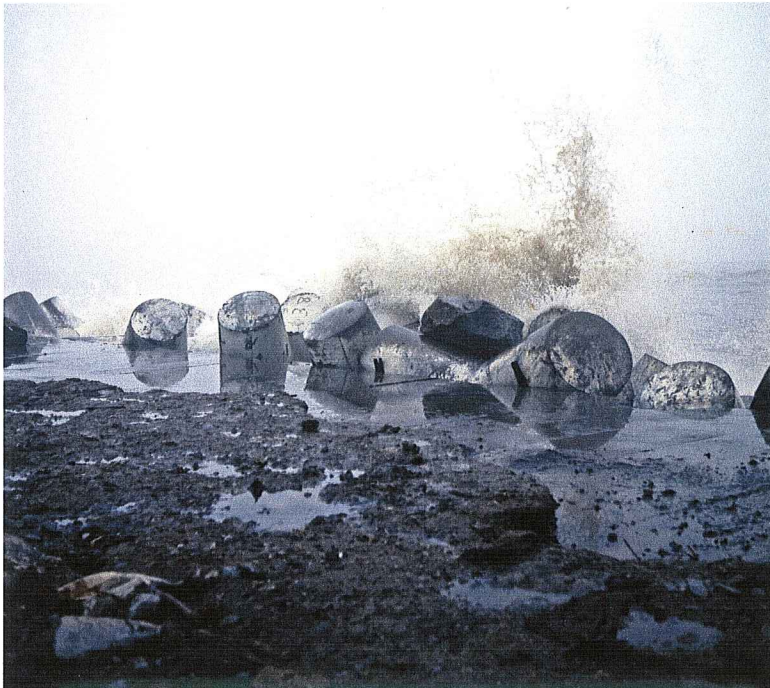
Figure 39. During a storm.
