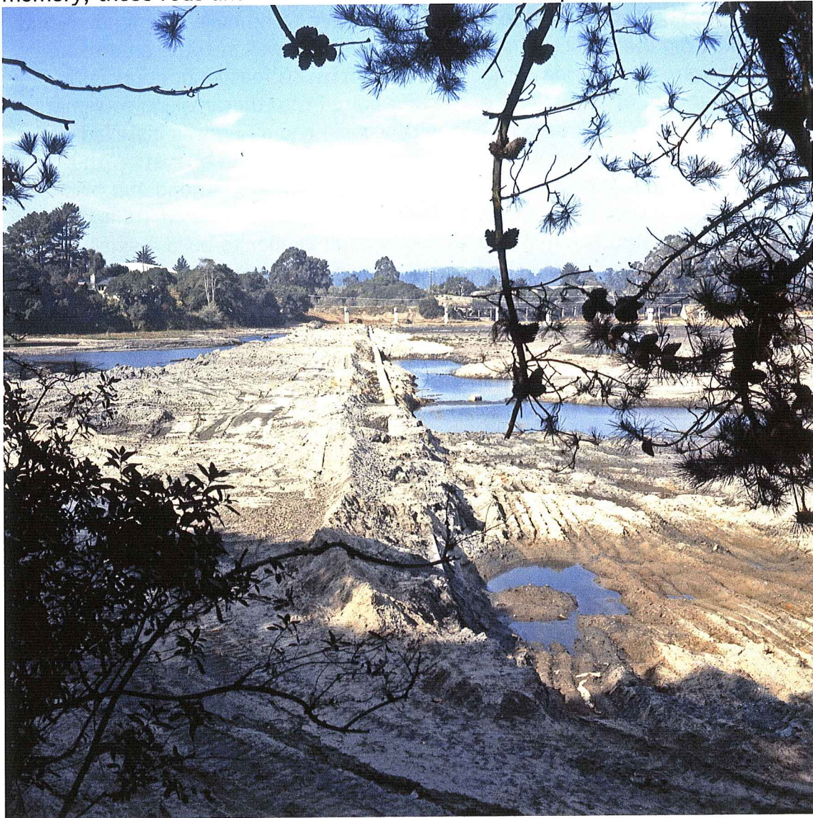
Figure 47. Top of a completed Bulkhead Wall. Before the damage. Facing north.
