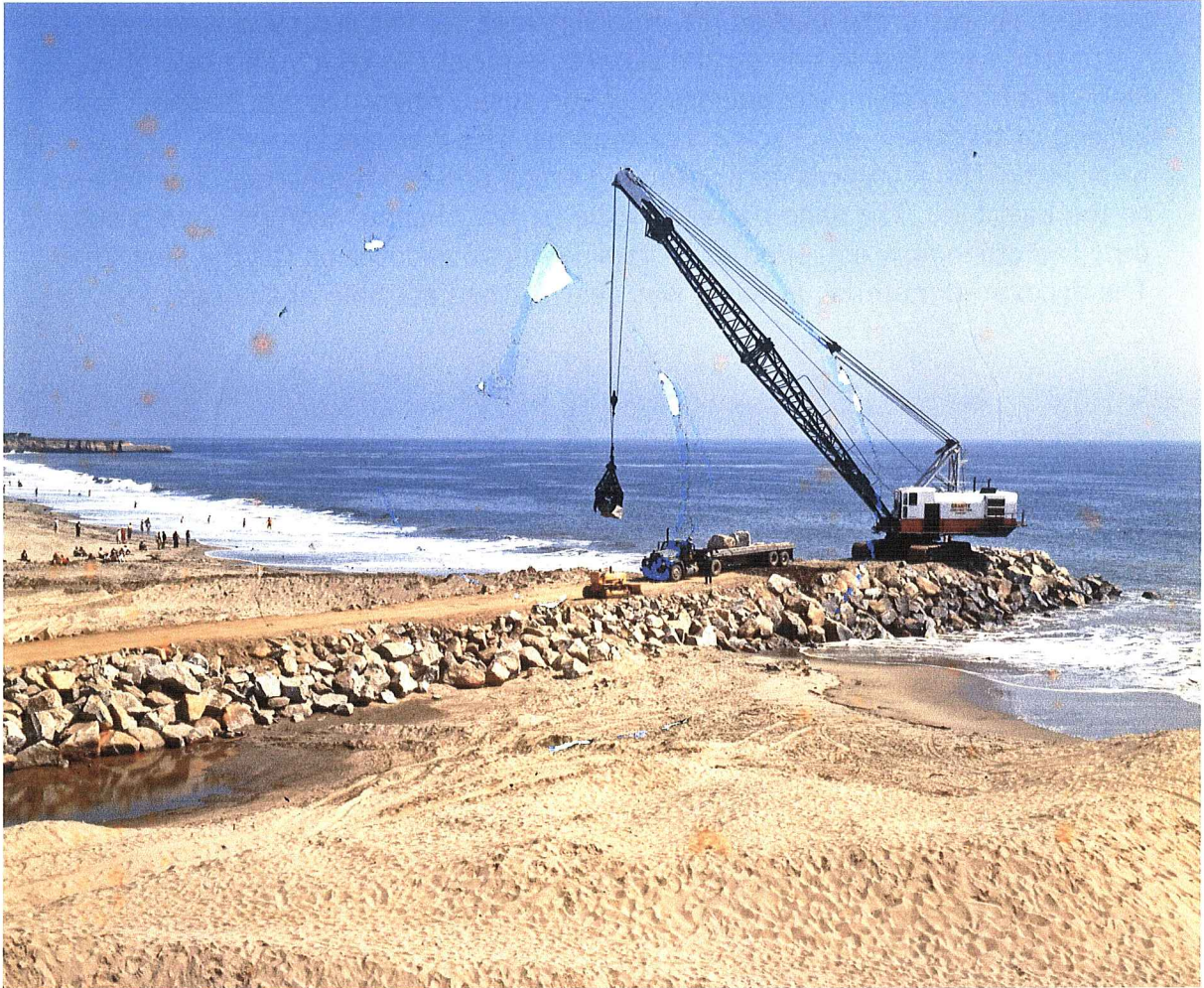
Figure 38. Crane on the East Jetty
