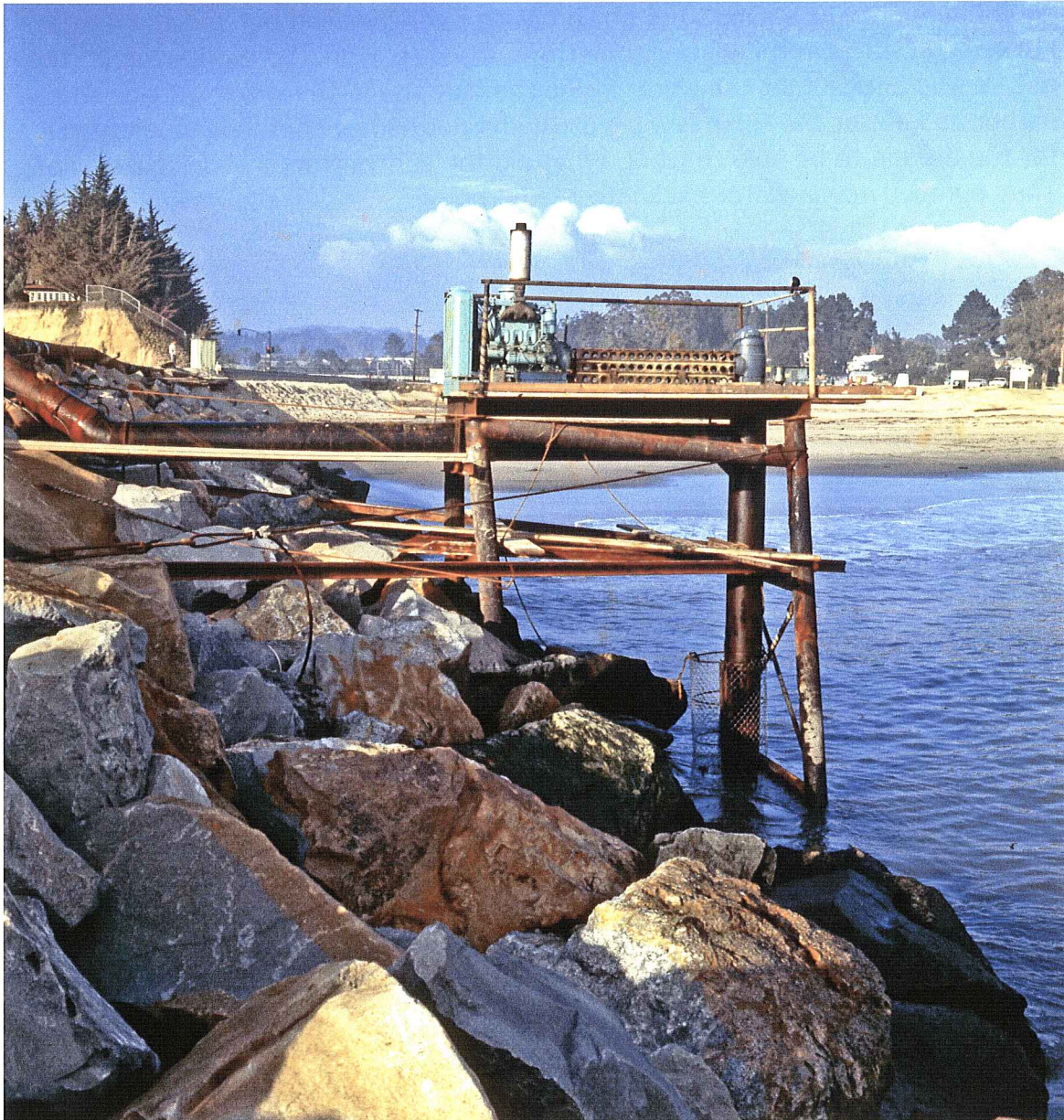
Figure 57. Set up installed to pump ocean water back into the harbor
