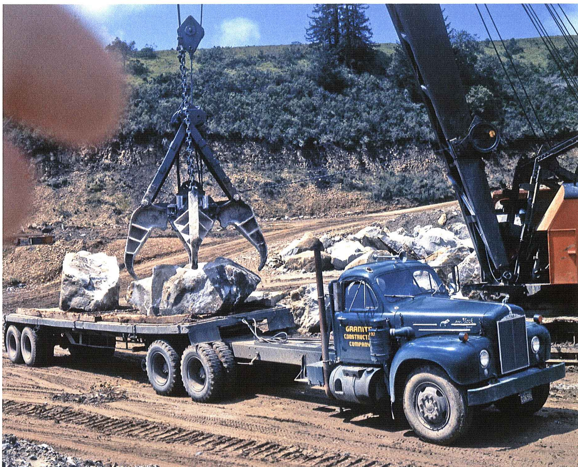
Figure 14. Loading an "A" stone in the quarry, 10 tons.
