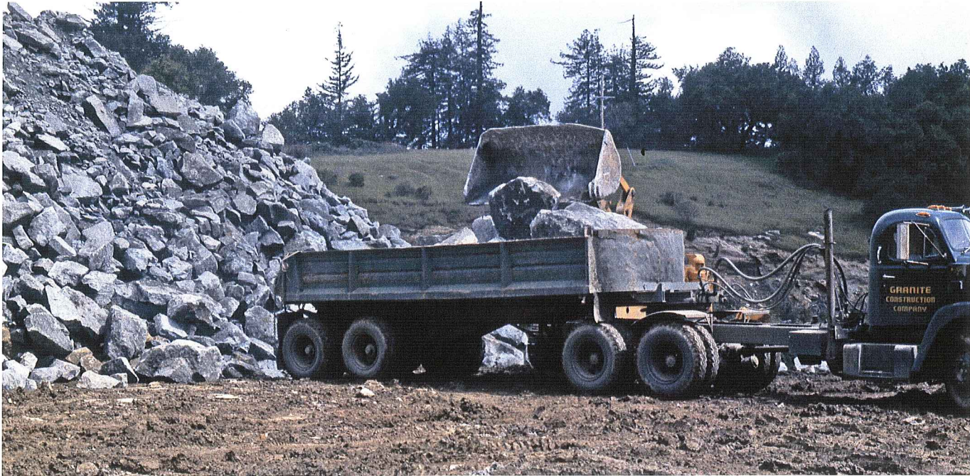
Figure 15. Loading "B2" stone, minimum 2 ½ to 3 1/2 tons each.
