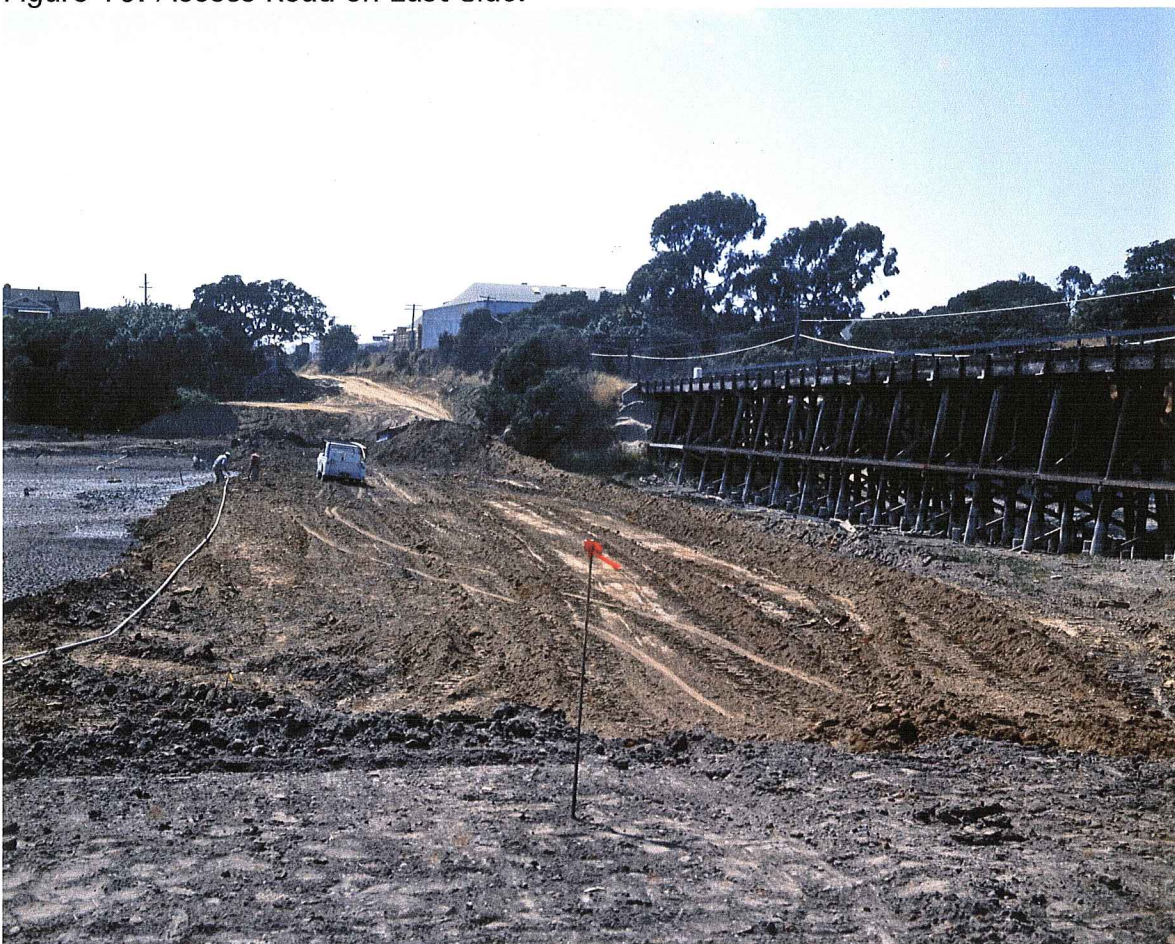
Figure 11. Access road & working pad for the Murray St. Bridge.
