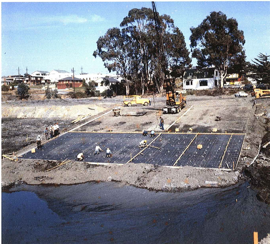
Figure 42. Installing reinforcing steel in launching ramp.
