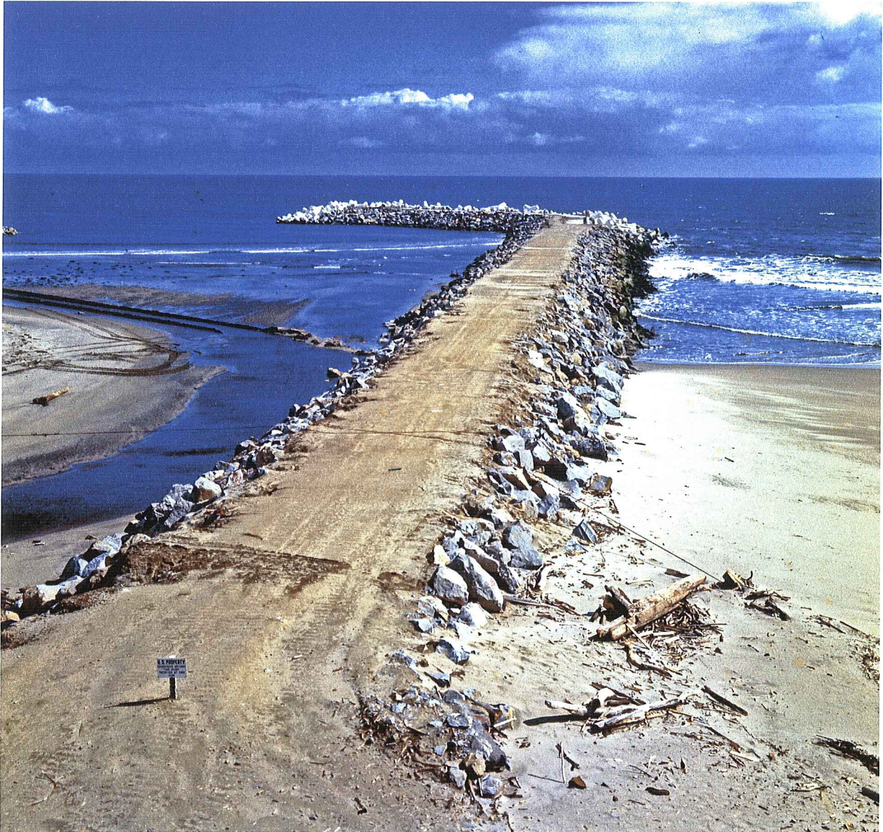
Fig. No. 5. West Jetty complete.
