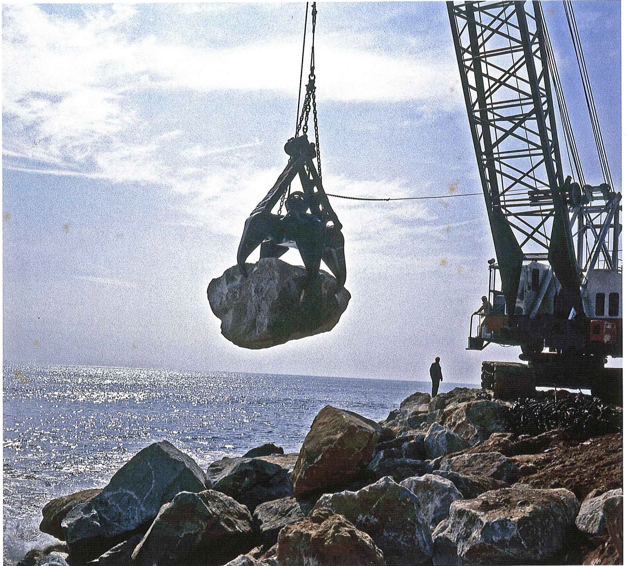
Figure: 29. Placing a 10-ton stone.
