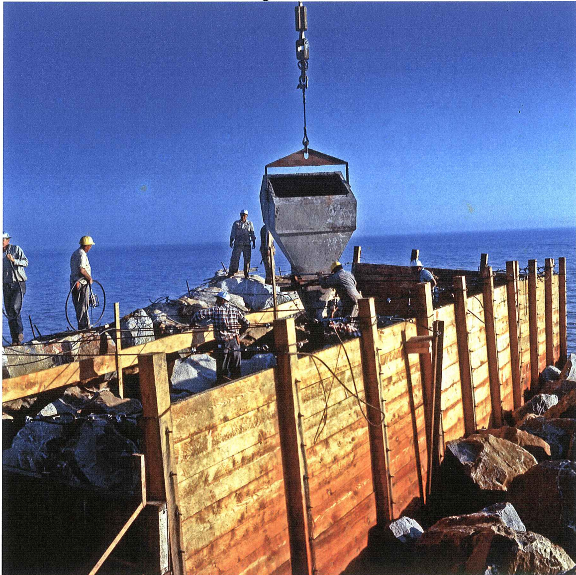
Figure: 26. Pouring grout into the spine forms
