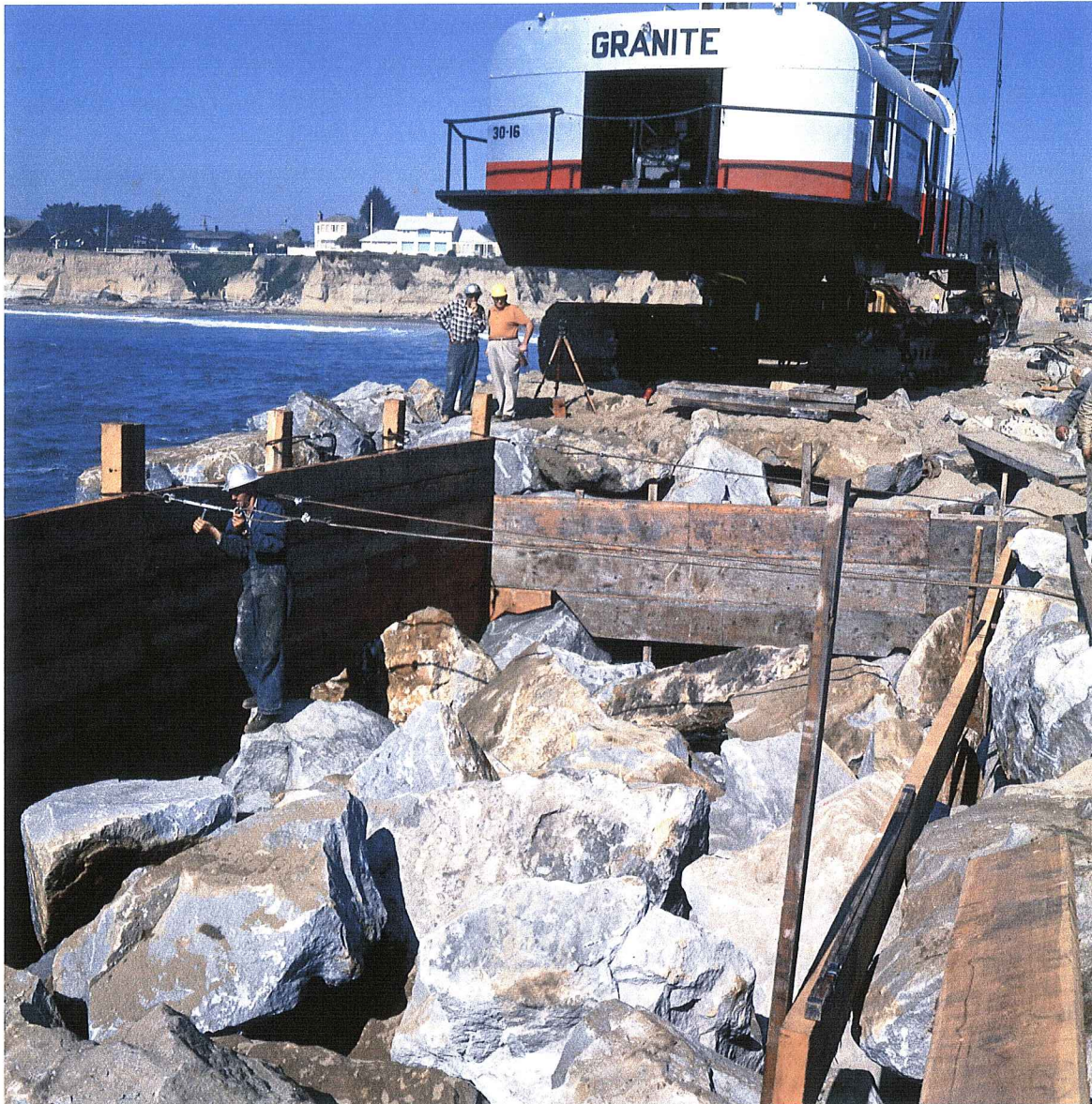
Figure: 27. Spine forms ready to receive concrete grout
