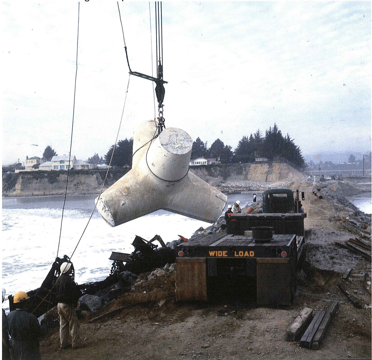
Figure 36. Unloading a Tetrapod.
