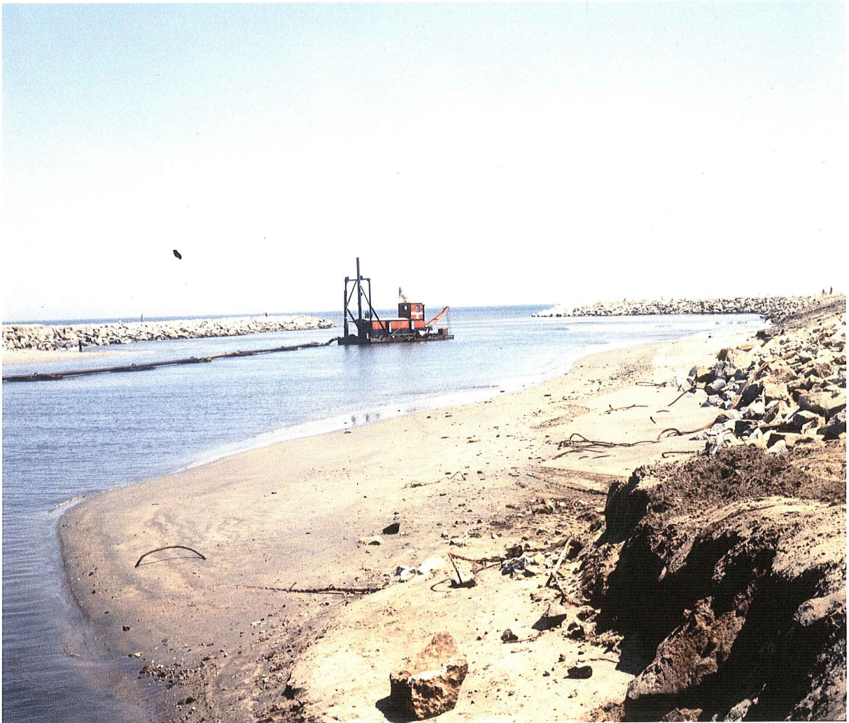
Fig. No. 10. Completing the opening, through the breakers.
