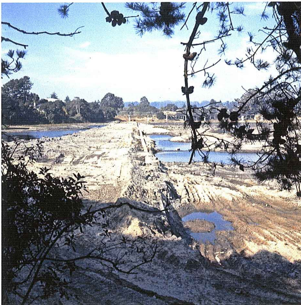
Figure 49. Top of capped bulkhead before damage.
