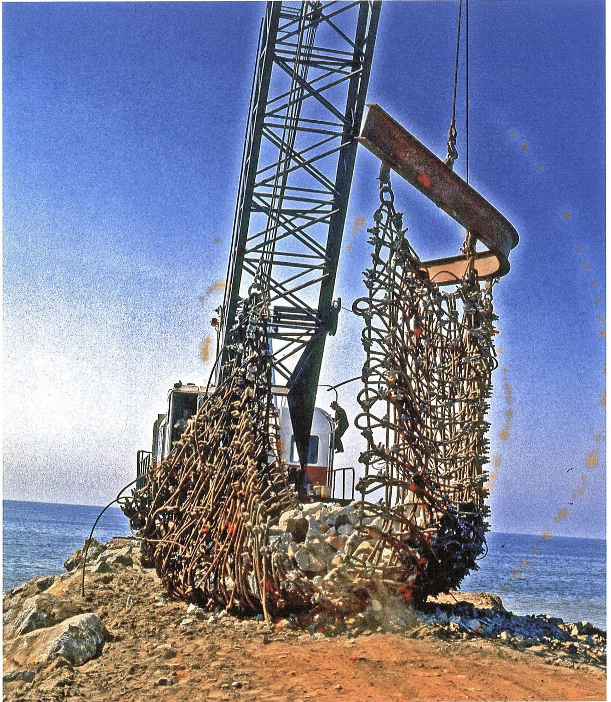
Figure 22. The net picking up a 20-ton load of quarry run material.
