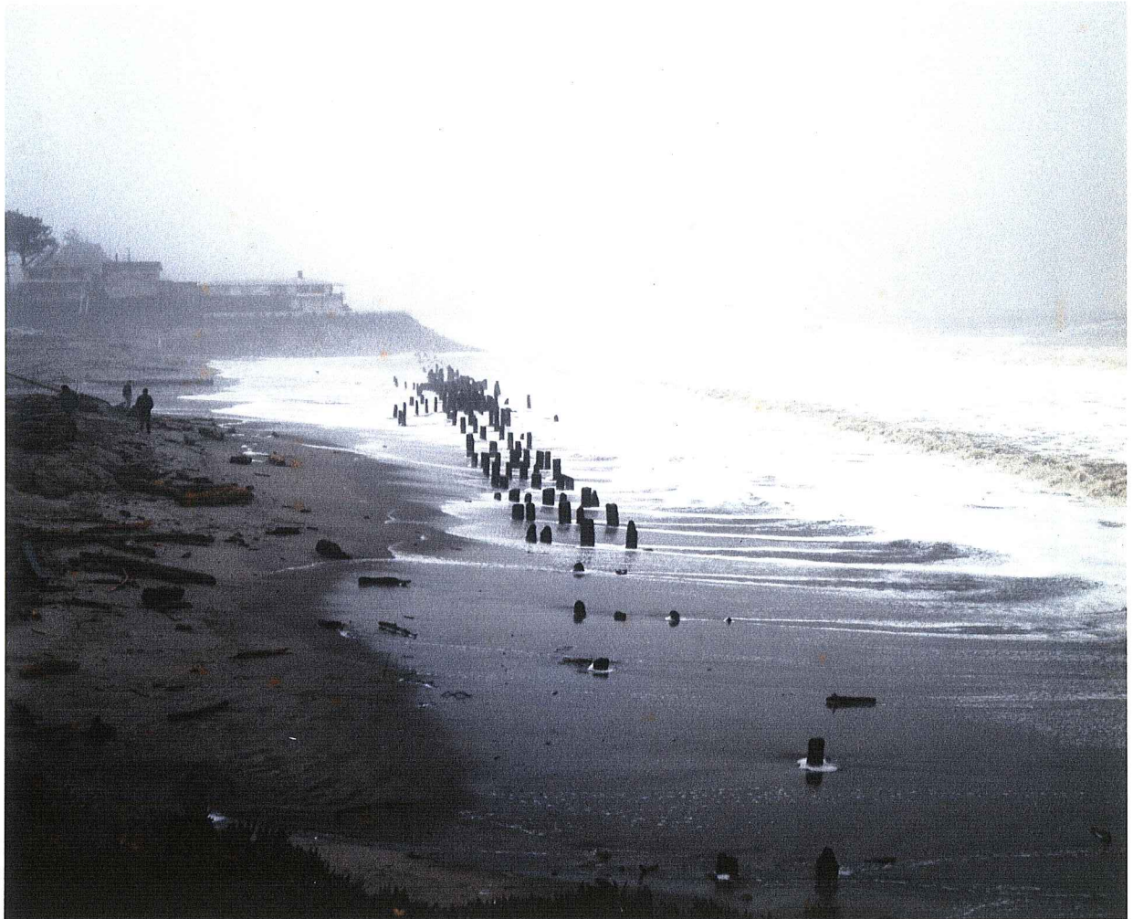
Fig. No 4. Pile trestle, remnants of Ocean Shore R.R. uncovered by the storm.
