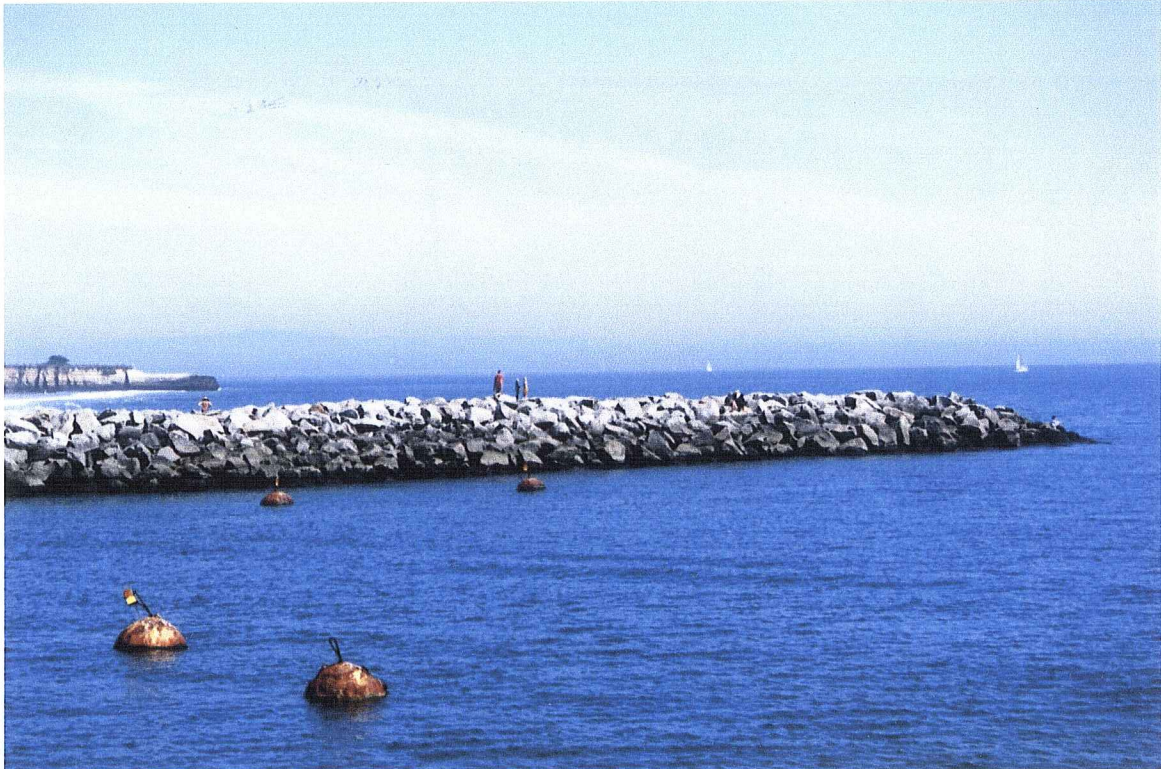
Figure 38a. Finished East Jetty. Harbor opening, notice buoys outlining channel.
