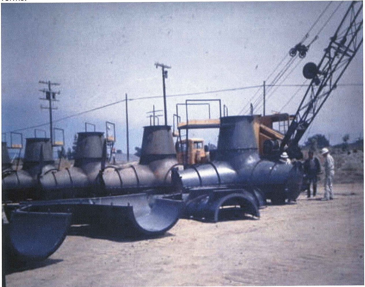
Figure 31. Set up to pour the first 8 tetrapods.
