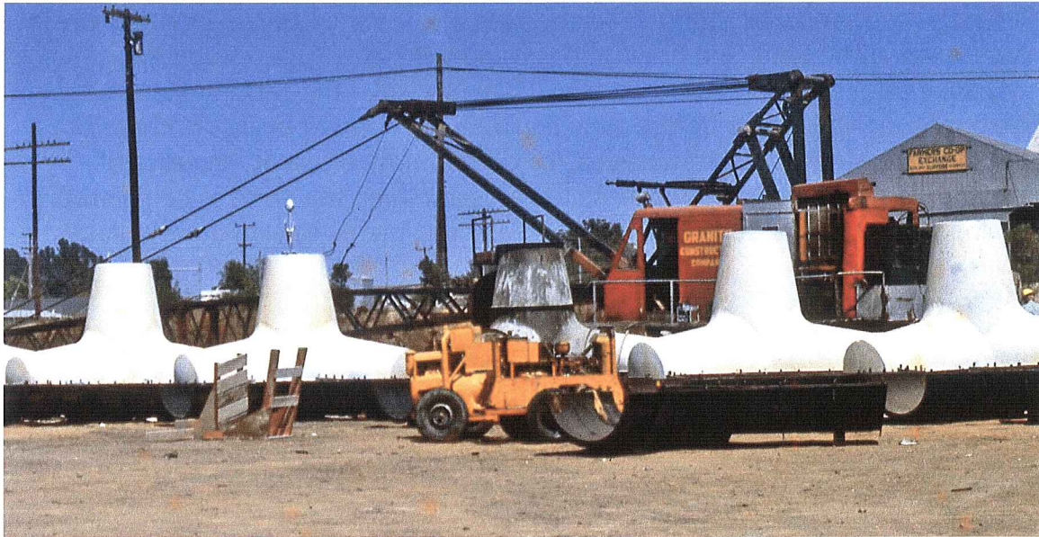
Figure 32: Removing tetrapods from bottom forms.
