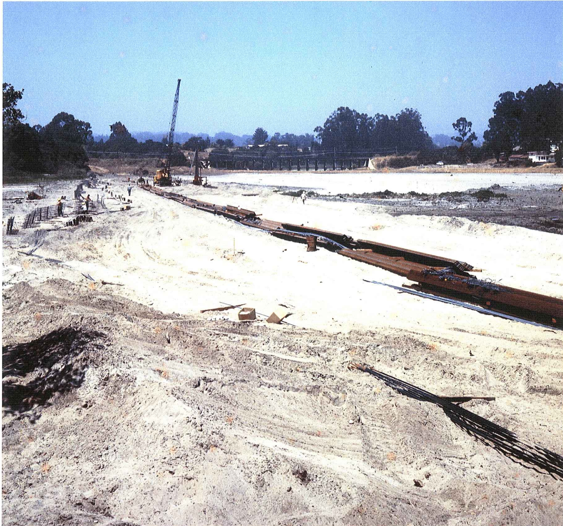
Figure 44. Laying out Sheetpiles for West Bulkhead.
