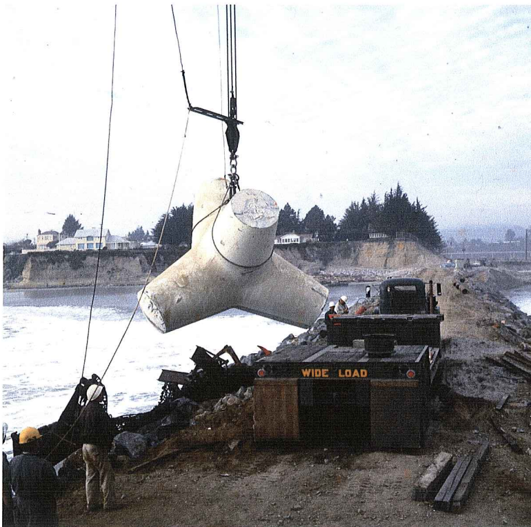
Figure 36. Unloading the first tetrapod.
