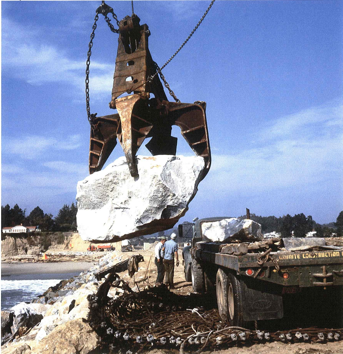
Figure: 28. Placing a 12 ton stone.
