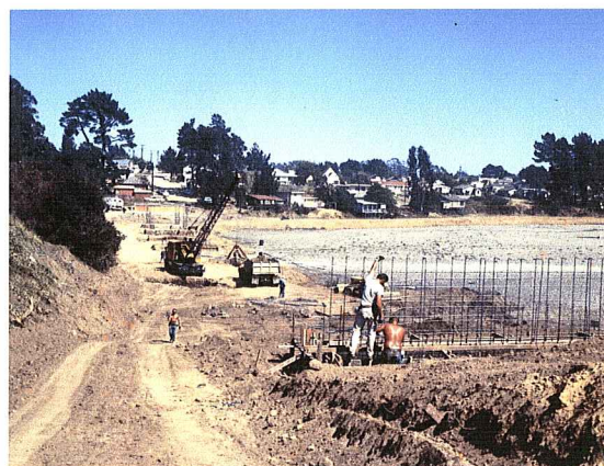
Figure 60. Installing reinforcing steel in piers for the Murray St. bridge.
