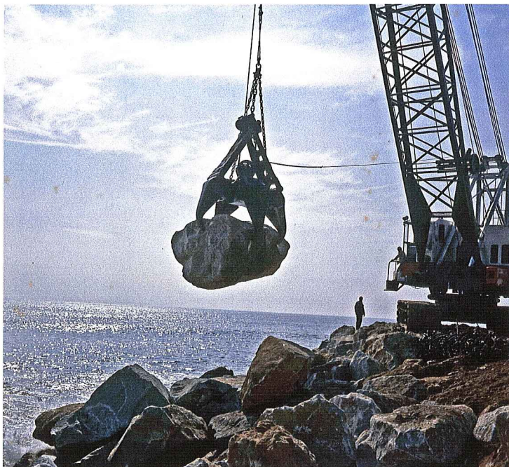
Figure 29. Crane unloading a 10-ton stone. Before the west jetty is complete.
