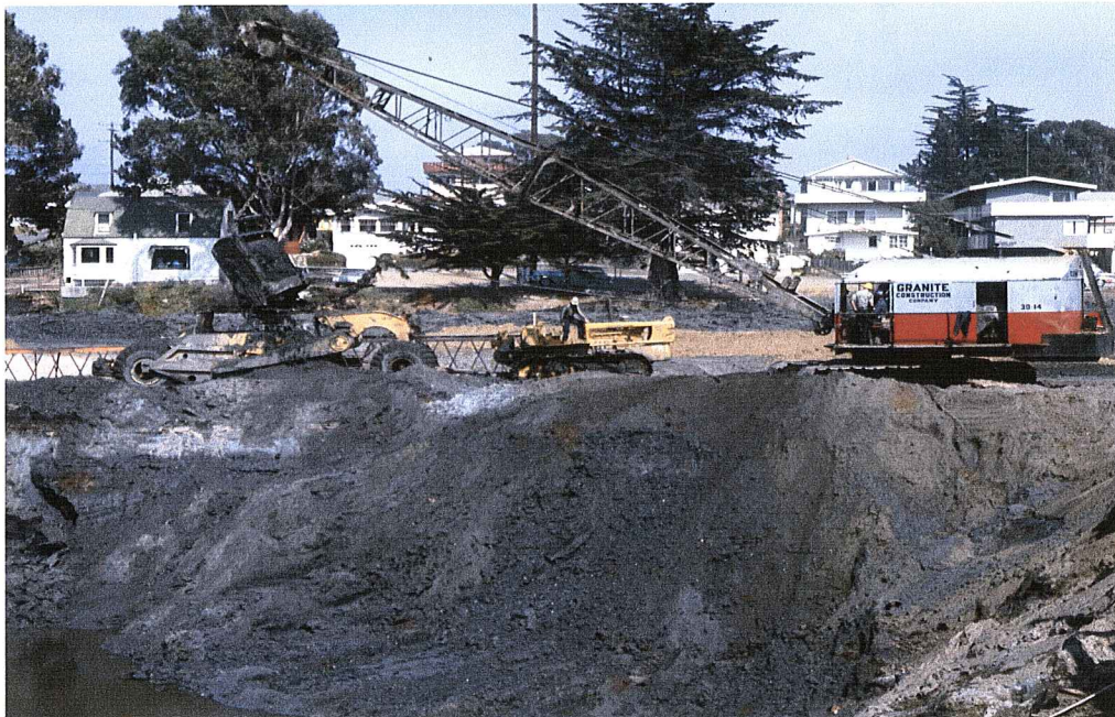
Figure 12. Beginning excavation for west jetty. Near present-day Aldo's.
