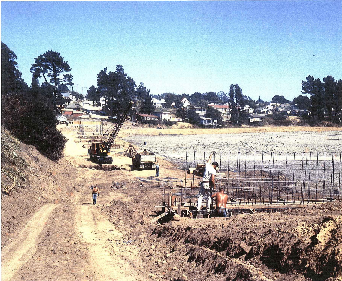
Figure 60. Installing reinforcing steel for Murray St. Bridge piers.
