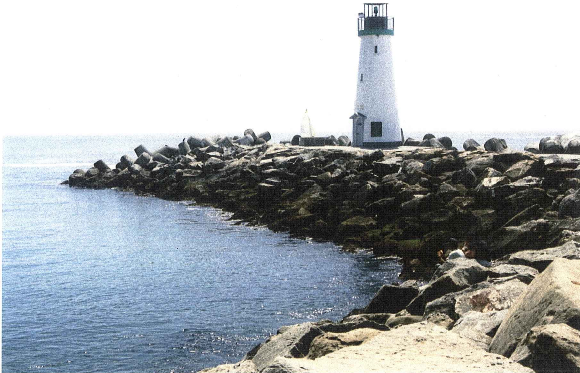
Figure 40a. Southerly half of the west jetty after completion
