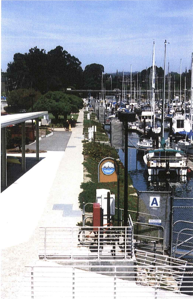
Figure 49a. Location of the completed bulkhead wall, present day. Facing North.
