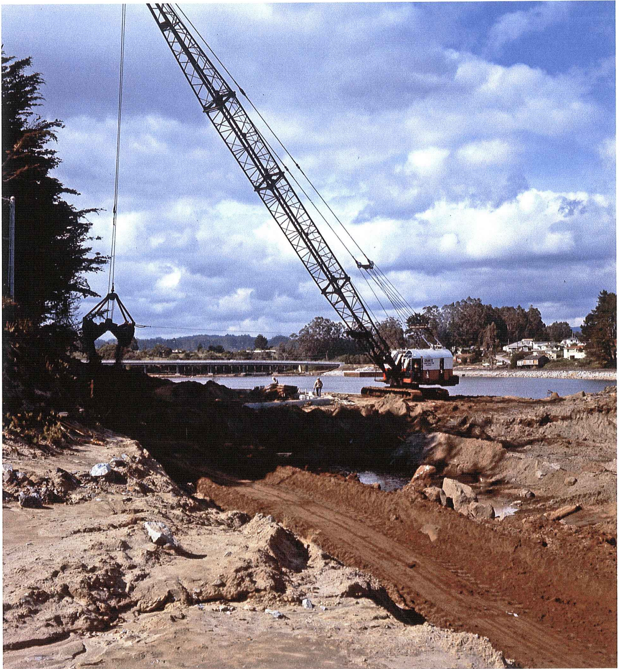
Figure 13. Excavating the cut in the bank for beginning the west jetty.
