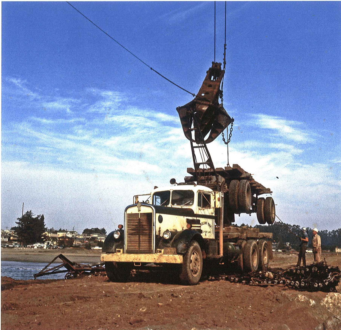
Figure: 21. Loading a trailer of a double truck & trailer unit onto the truck to back off the jetty. A truck & trailer unit cannot turn around on the jetty.
