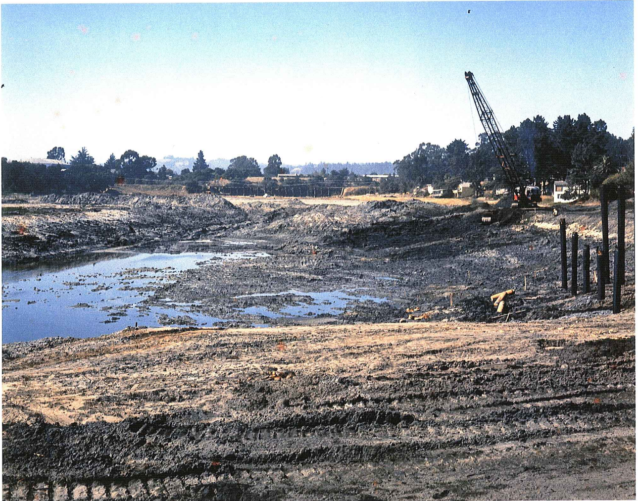
Figure 41. Crane with dragline bucket excavating Boat Launching Ramp
