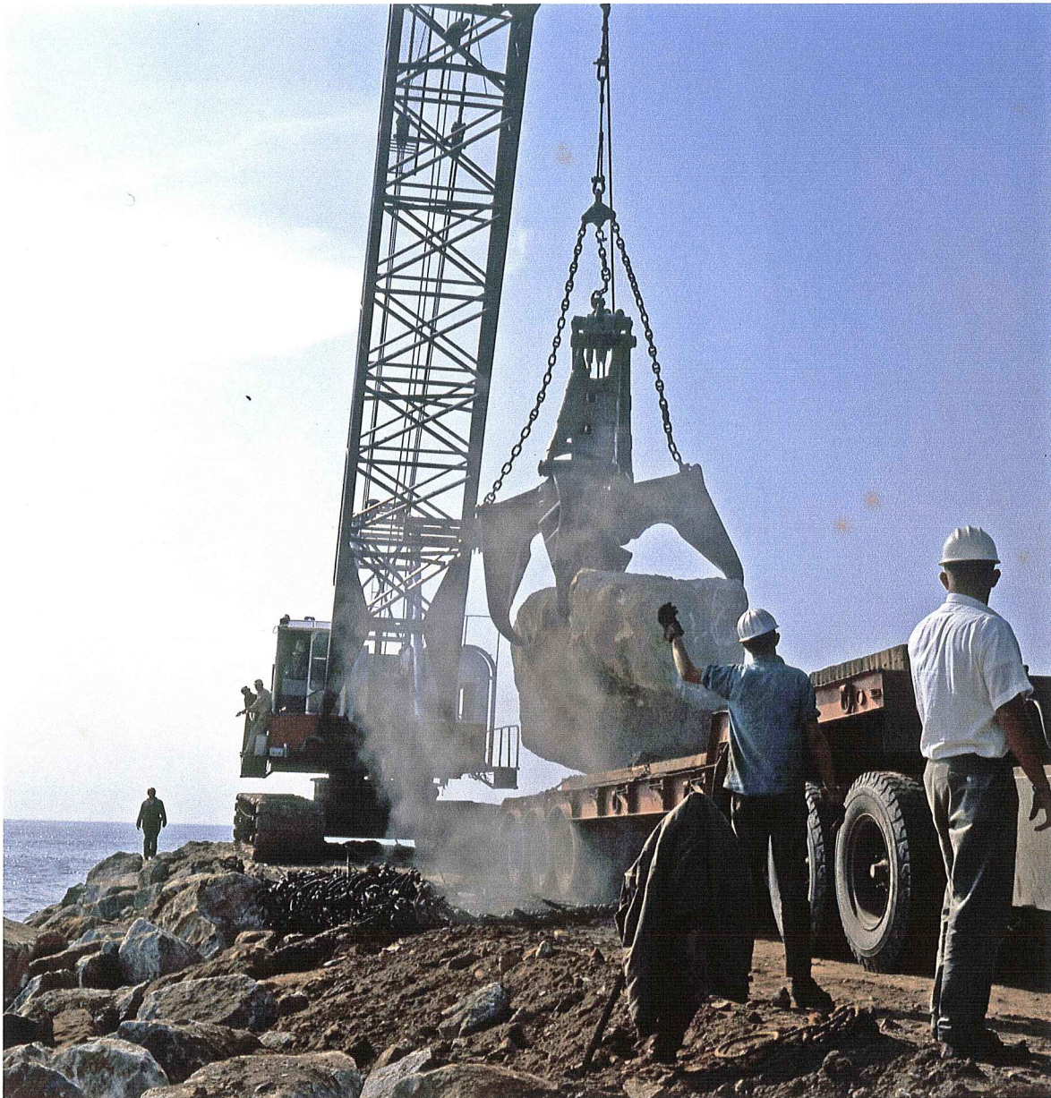
Figure: 19. Unloading an 18-ton stone. The largest stone in the jetty.
