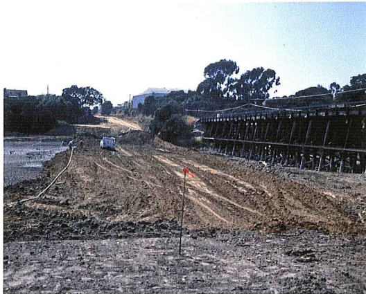
Figure 11. Access road and working pad for Murray St bridge.
