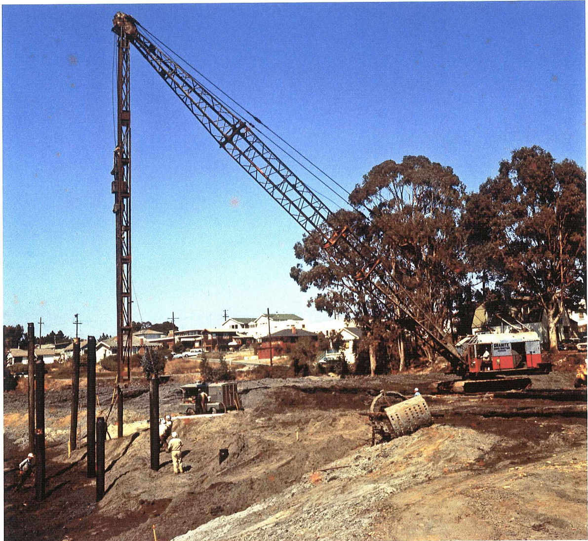
Figure 43. Driving foundation Piles for Boat Launching Ramp.
