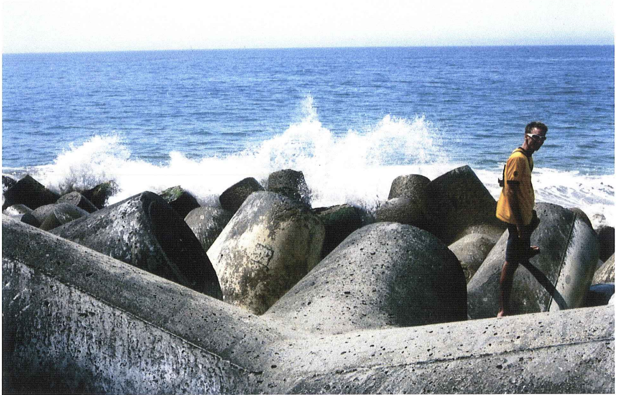
Figure 39a. A pile of tetrapods.
