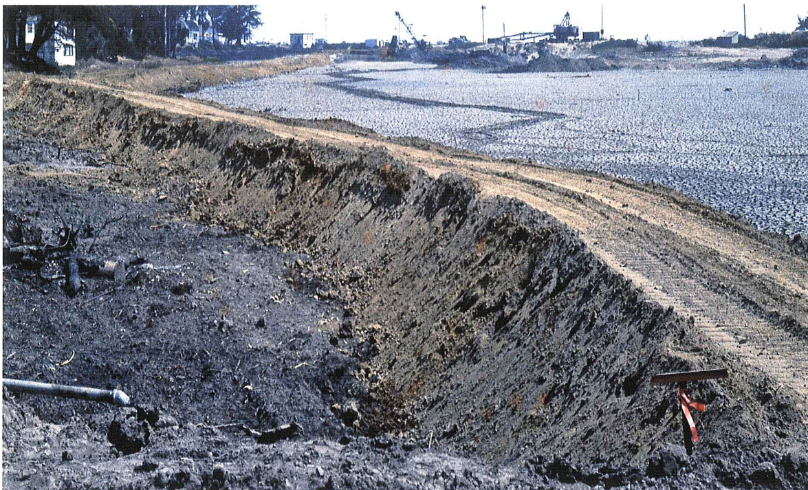
Figure 10. Access Road on East Side.
