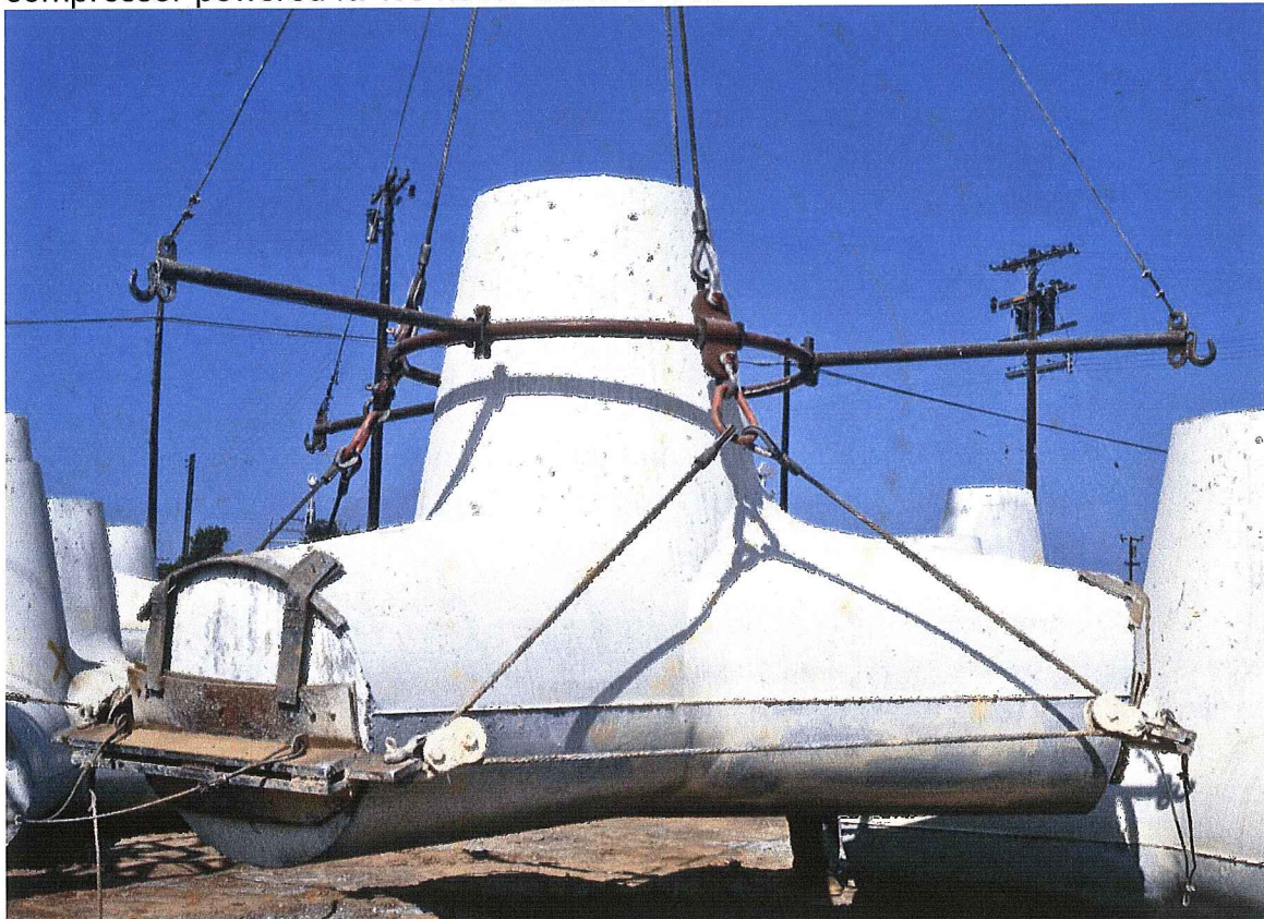
Figure 34. A tetrapod in its carrying sling.
