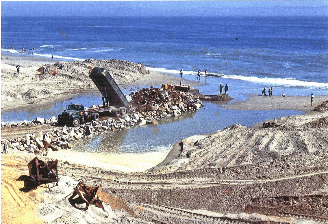
Figure 18. Dumping and placing rock on the west jetty
