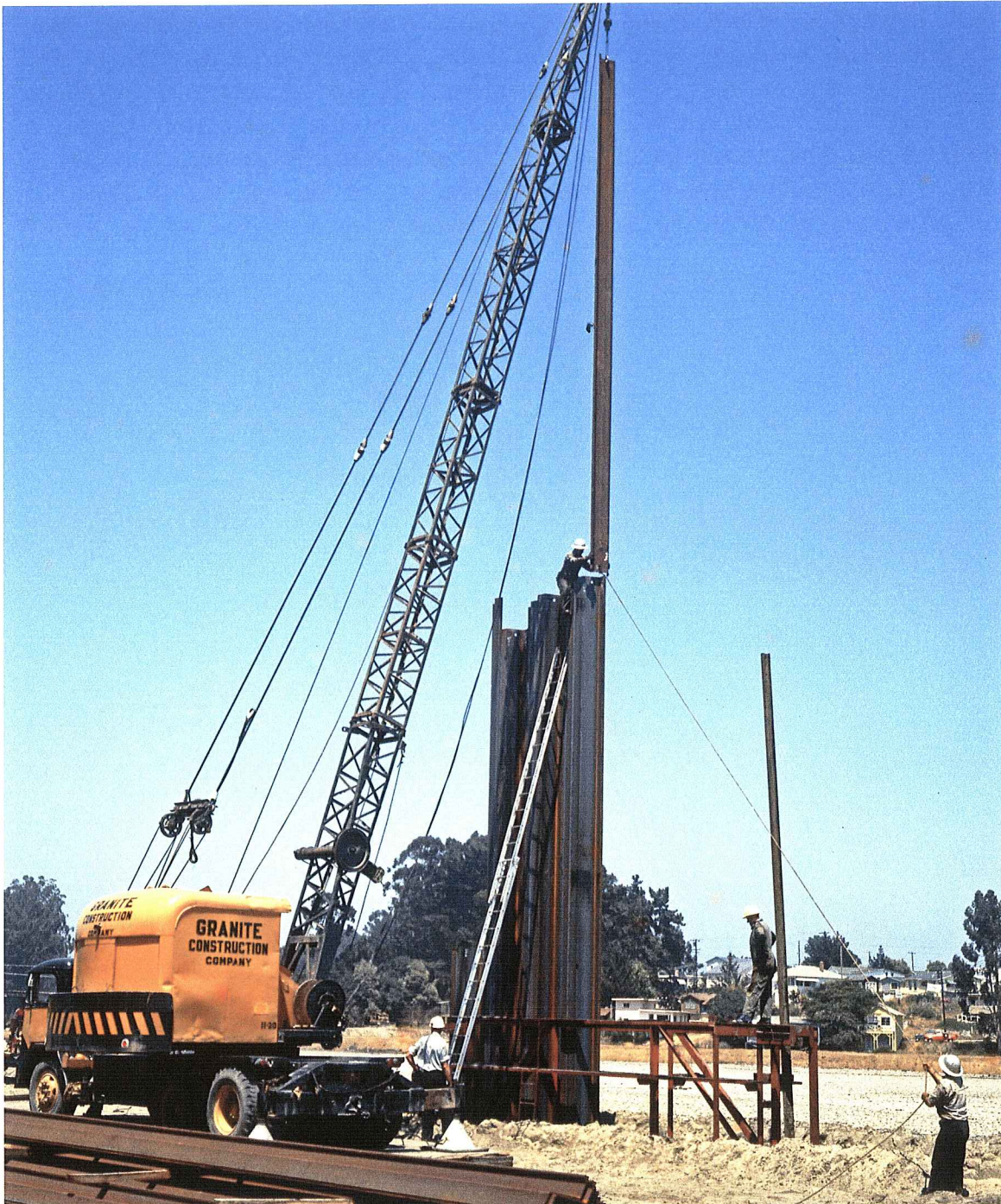
Figure 45. Beginning to drive sheet piles for the west bulkhead.
