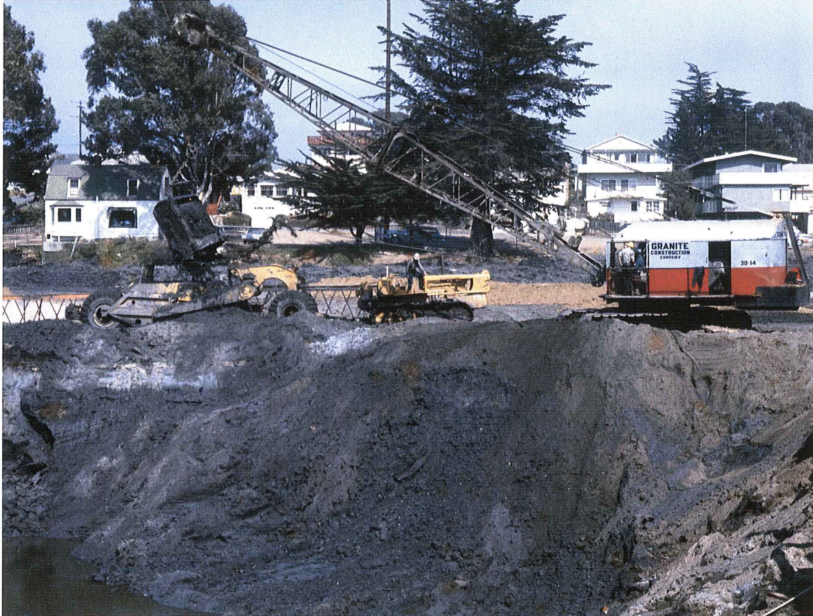
Figure 12. Excavating for the start of construction for the West jetty.
