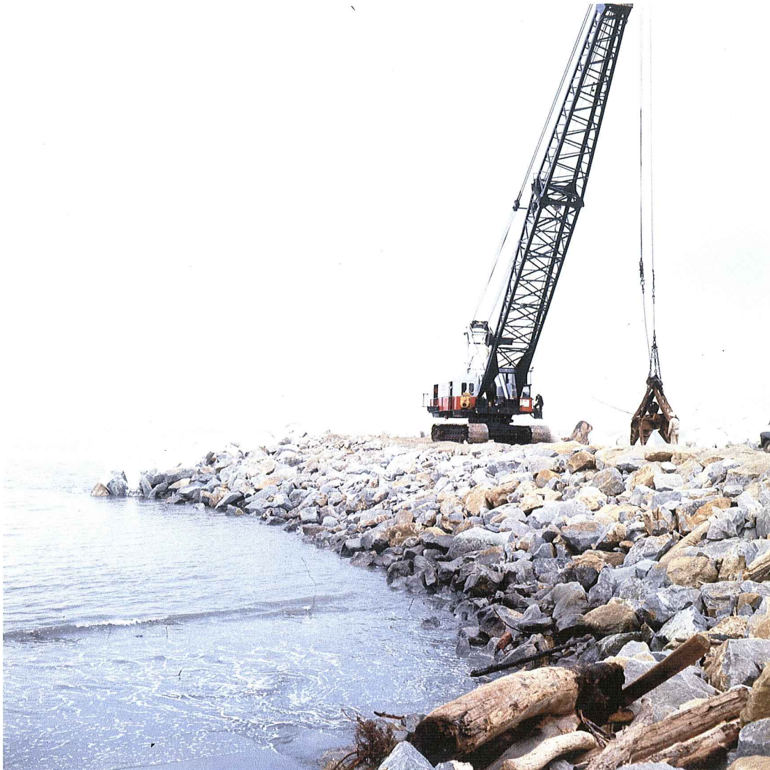
Figure 40. Crane completes the West Jetty.
