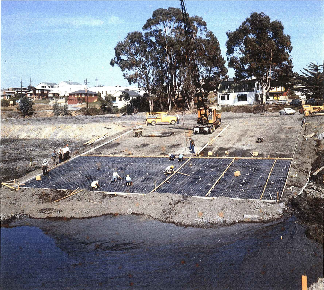
Figure 42. Installing reinforcing steel for the concrete launching ramp.
