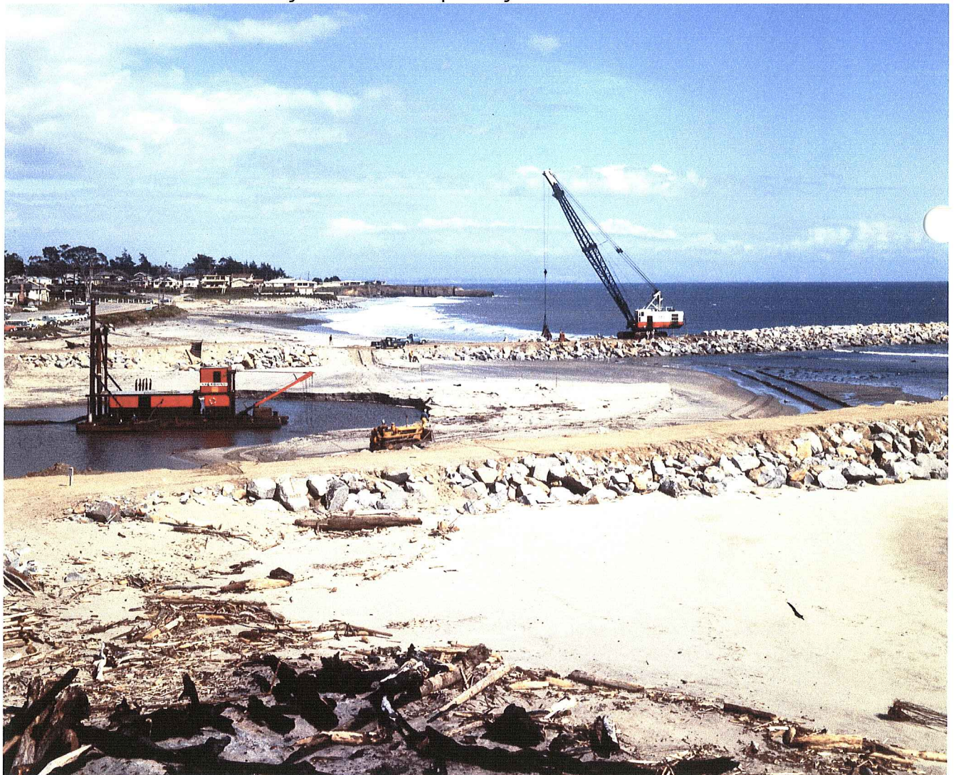
Figure 56. Dredging through for the harbor opening, the first time.
