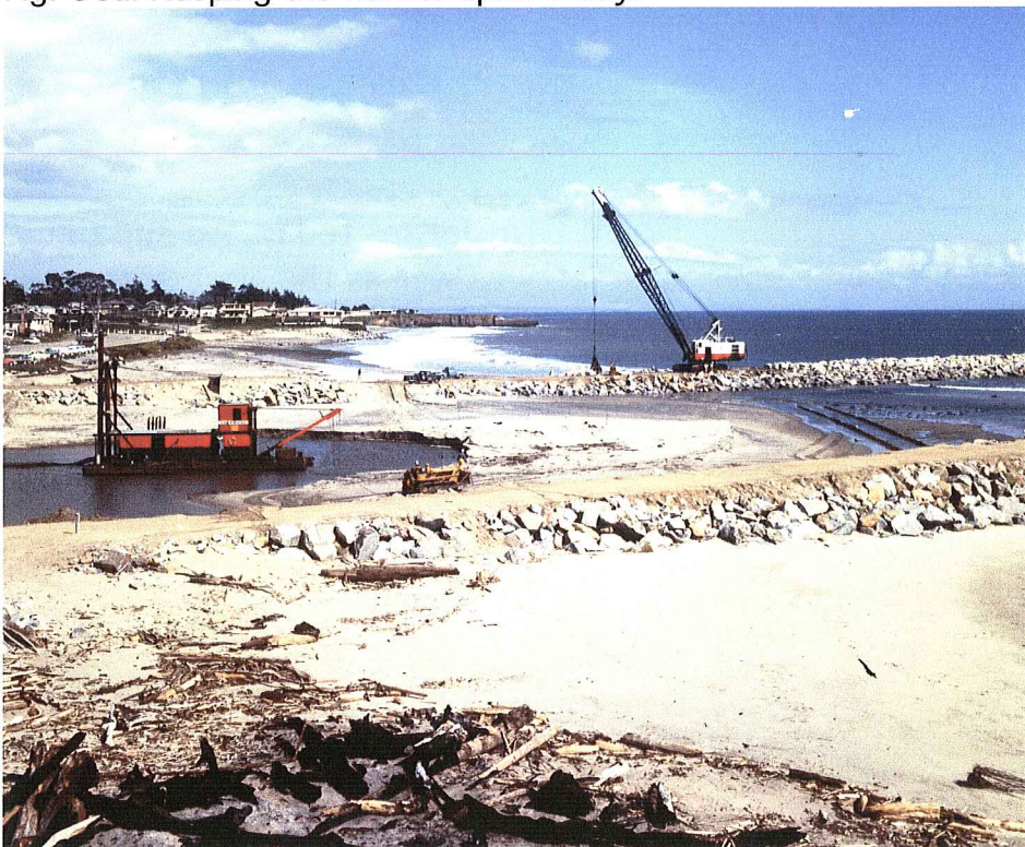
Figure 56. Dredging through the opening for the first time.
