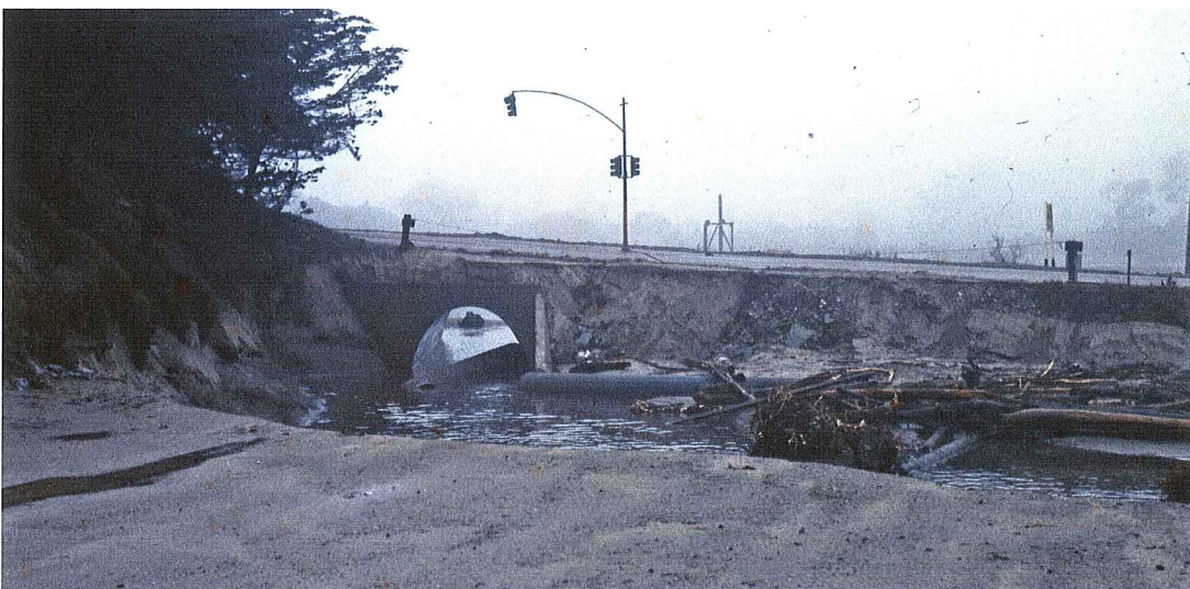
Figure 2. East Cliff Drive before the Harbor. Bridge is a Corrugated Metal Arch attached to a Concrete slab on footings, with headwalls.
