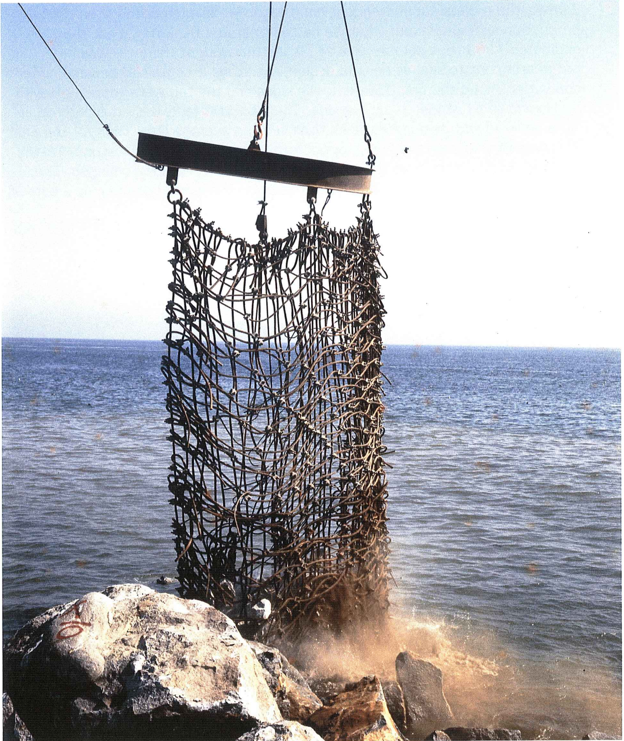
Figure: 24. The net dumping a load.
