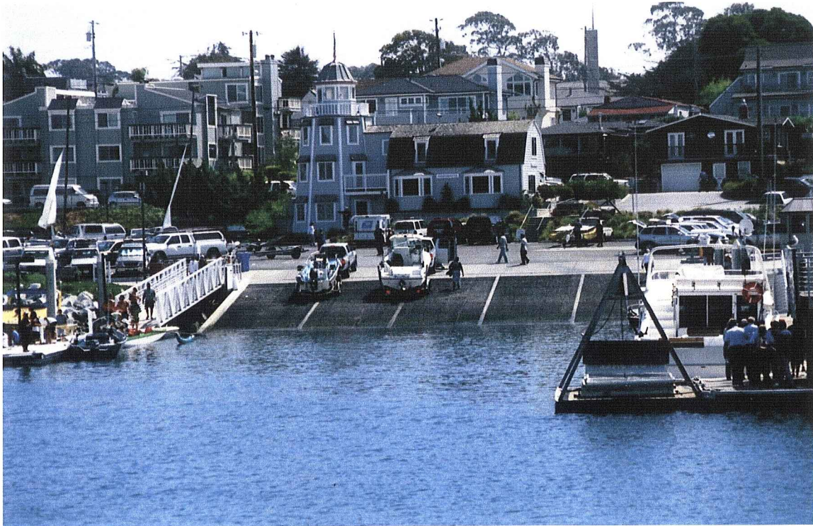
Figure 42a. Completed launching ramp.
