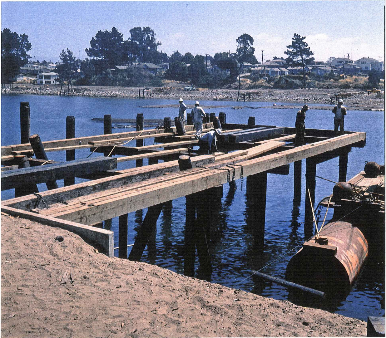
Figure 51. Installing Caps and Stringers for the public pier.
