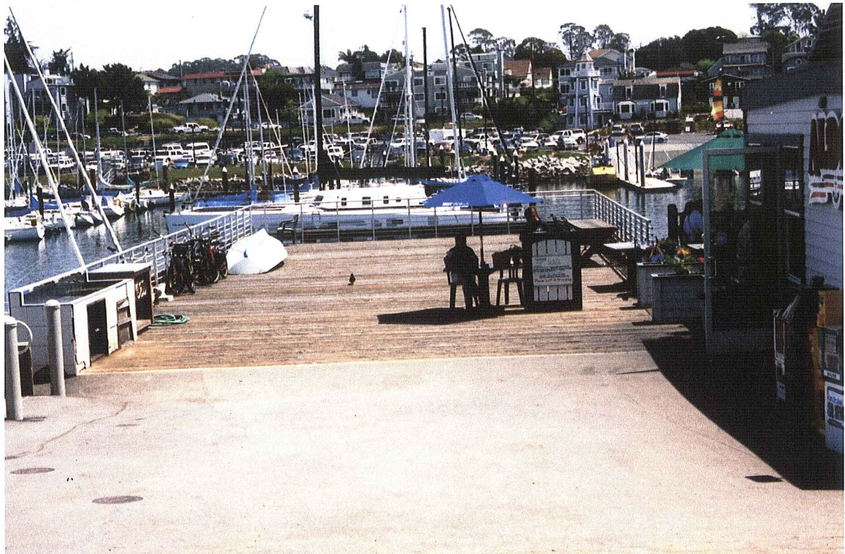
Figure 53a. Public pier near Aldos.
