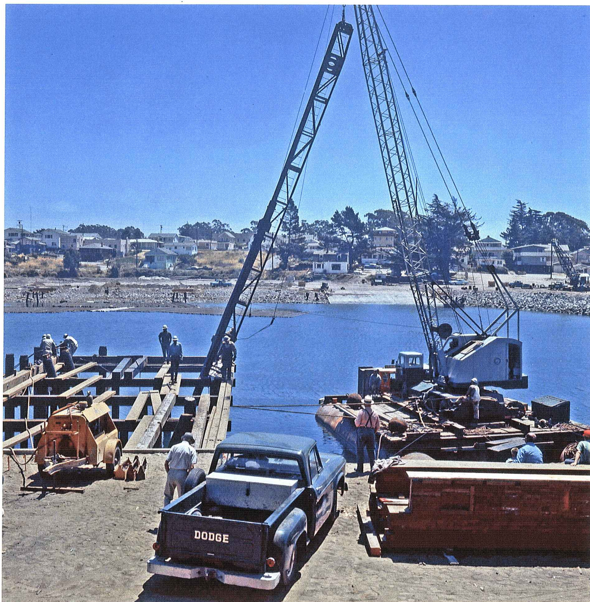
Figure 52. Constructing the Public Pier.
