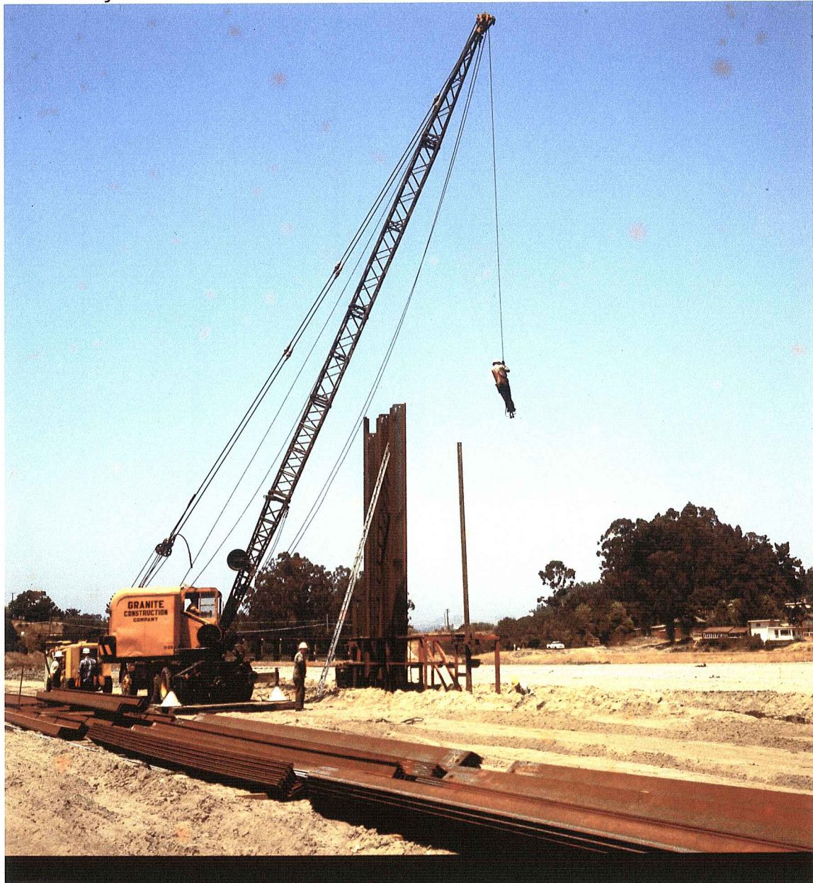
Figure 46. Driving Sheet piles for the West Bulkhead.
